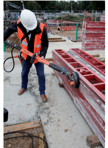
Cleaning shuttering segments in upright position
