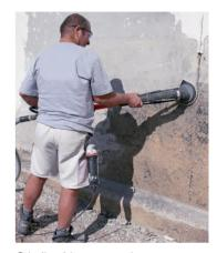
Grinding bitumen coating with PCD grinding disc
